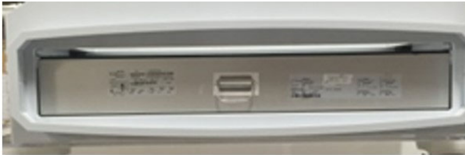
Primary filter fully seated to rear of BIBO housing
