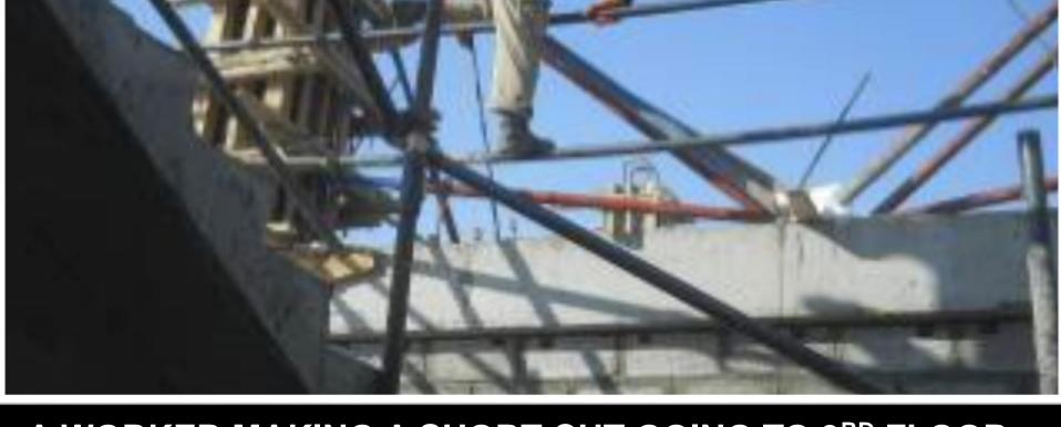
A WORKER MAKING A SHORT CUT GOING TO 3<sup>RD</sup> FLOOR LEVEL FROM 2<sup>ND</sup> TO 3<sup>RD</sup> FLOOR STAIRCASE
